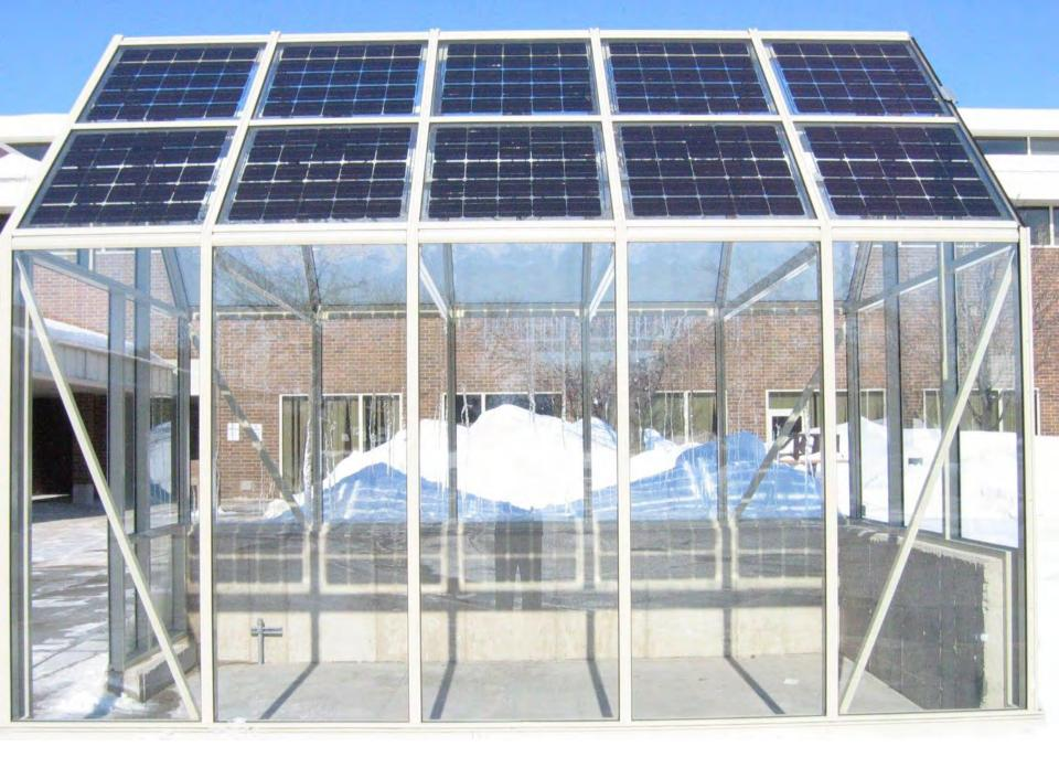
**Building Integrated Photovoltaic Bus Shelter – 1.0 kW (2007)**
